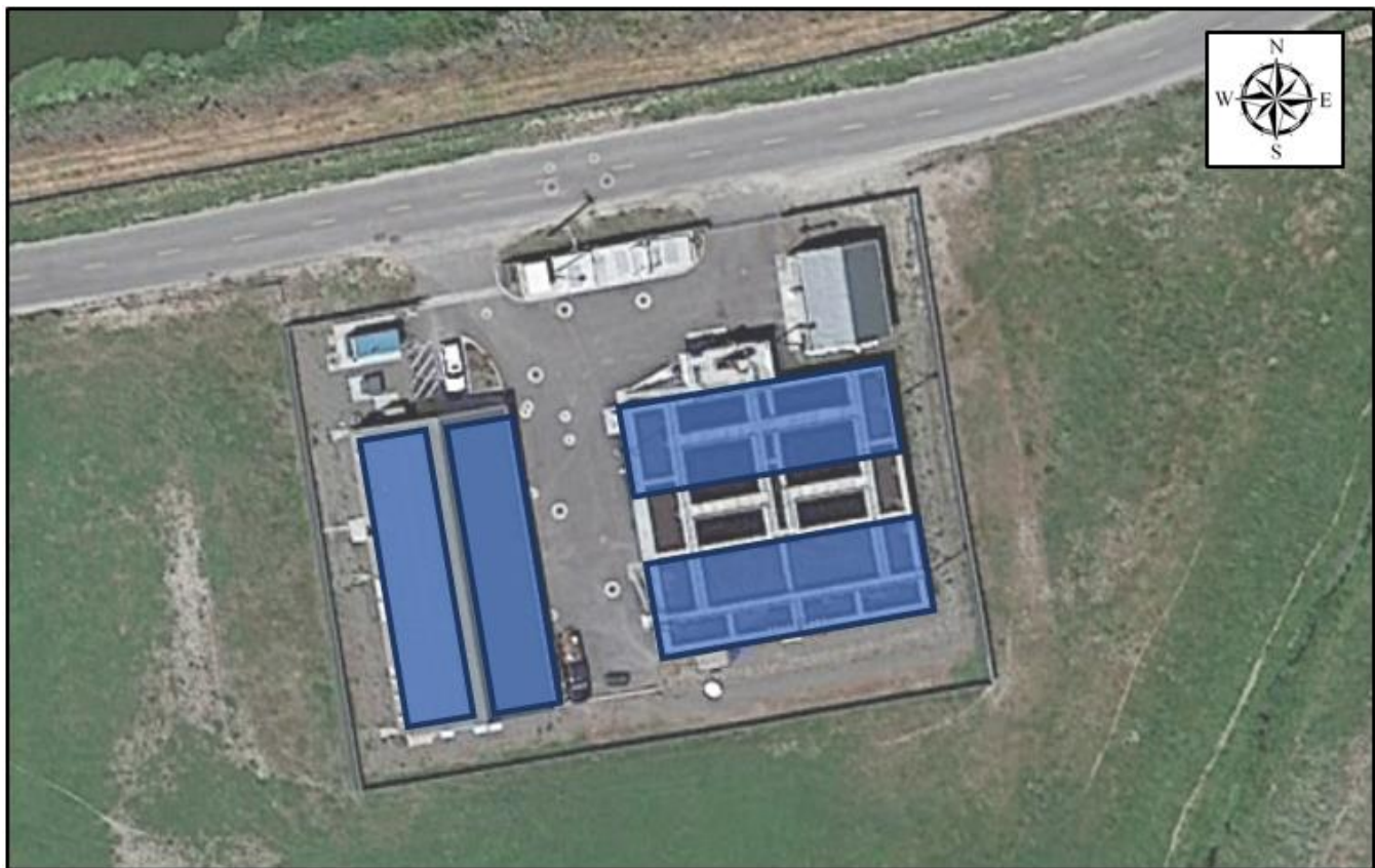
Figure 3 Available area for solar PV installation at the City of Ferndale’s WWTP.
