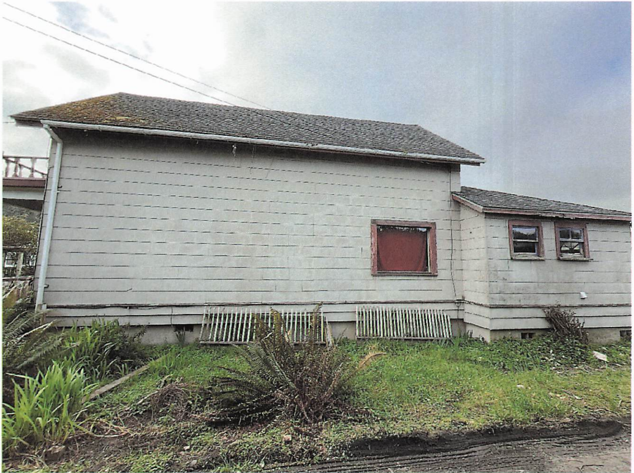
View of east side of existing house
