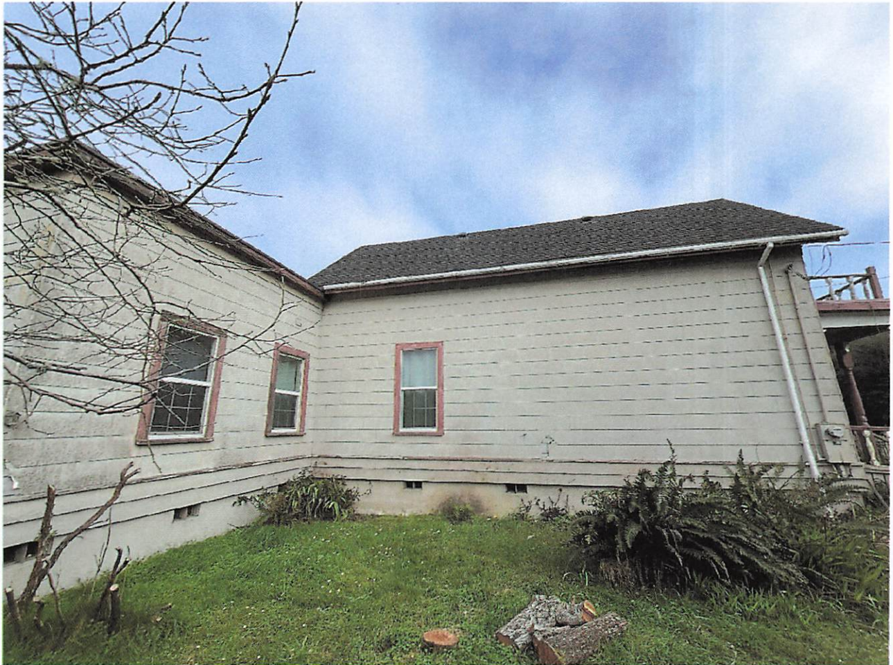
View of west side of existing house
