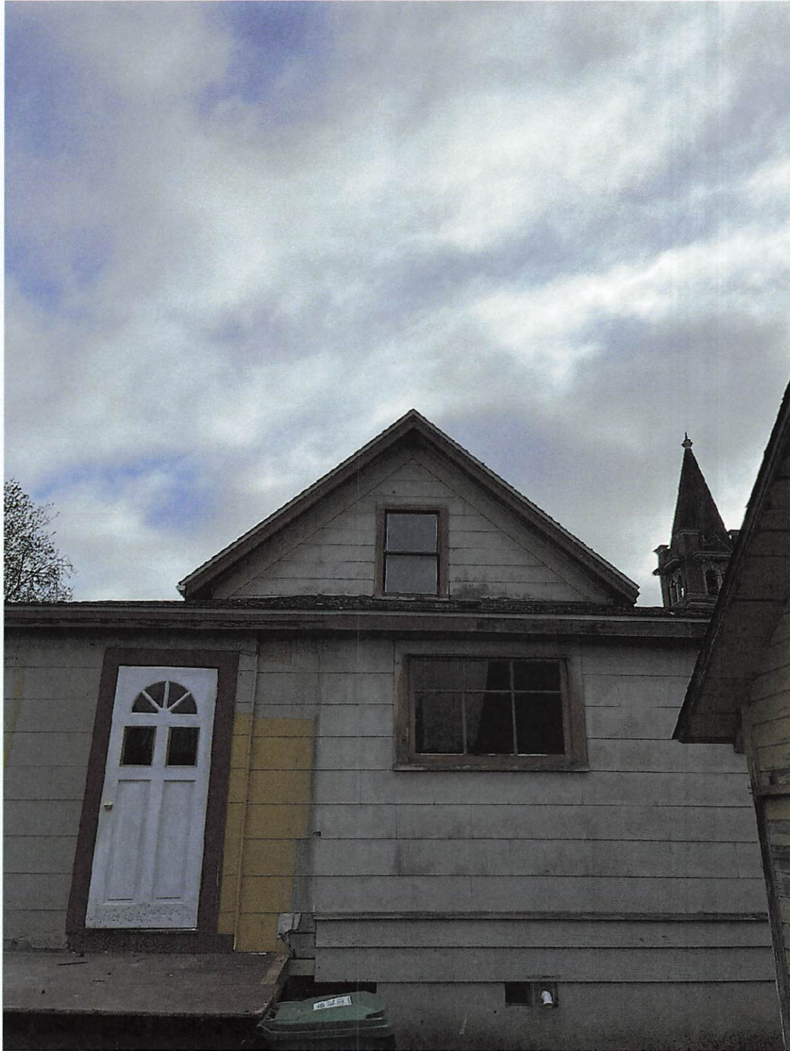
View of rear of existing house
