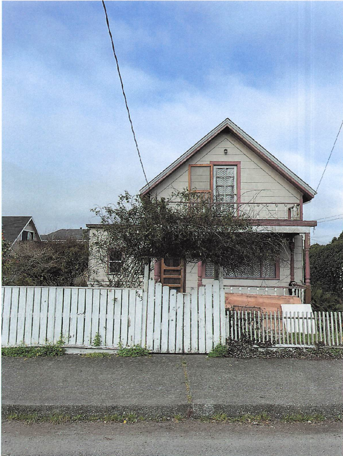
View of front of existing house
