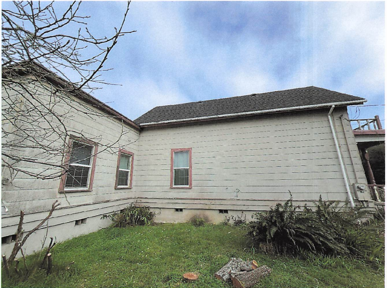
View of west side of existing house
