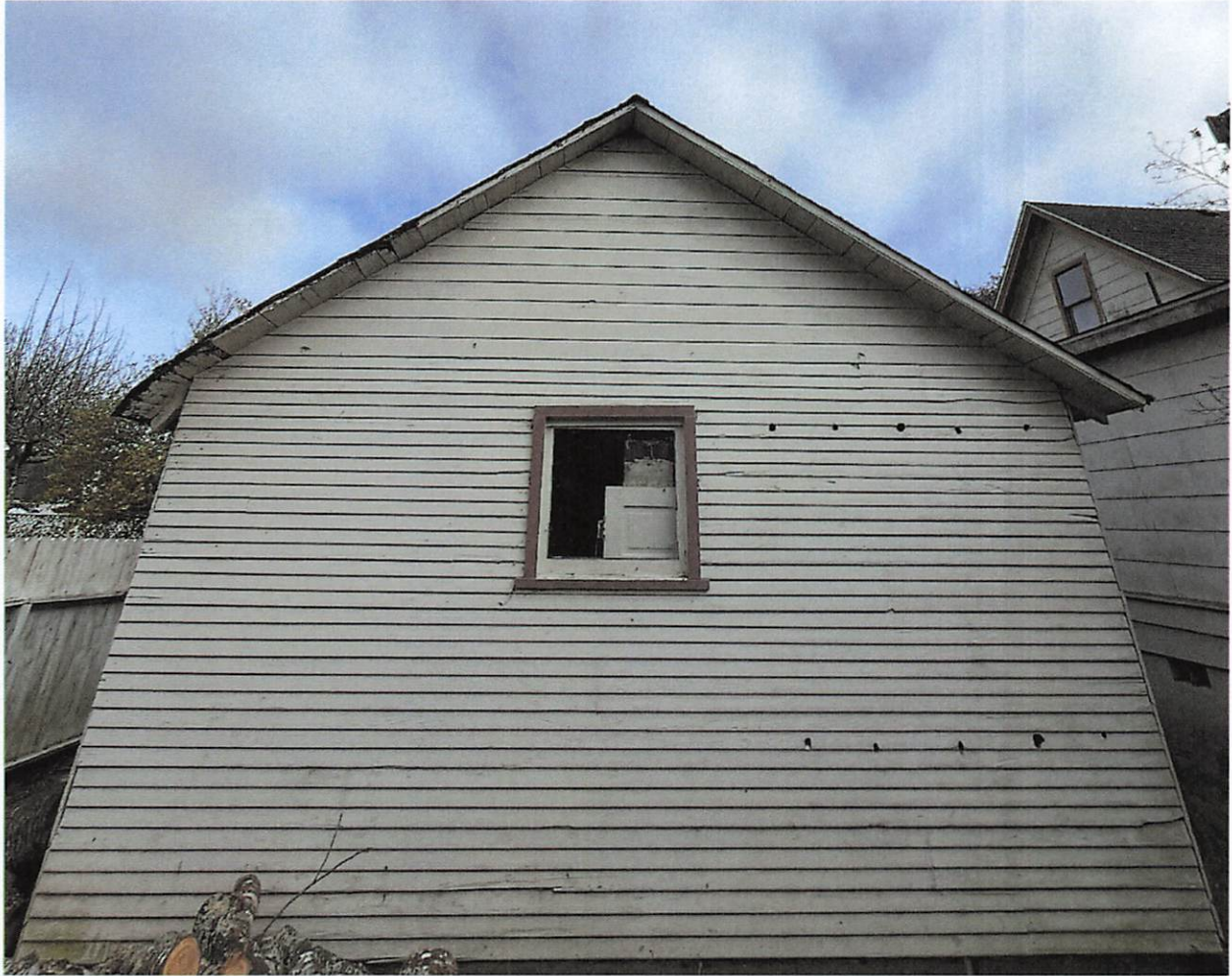
View of rear (west facing) of existing garage
