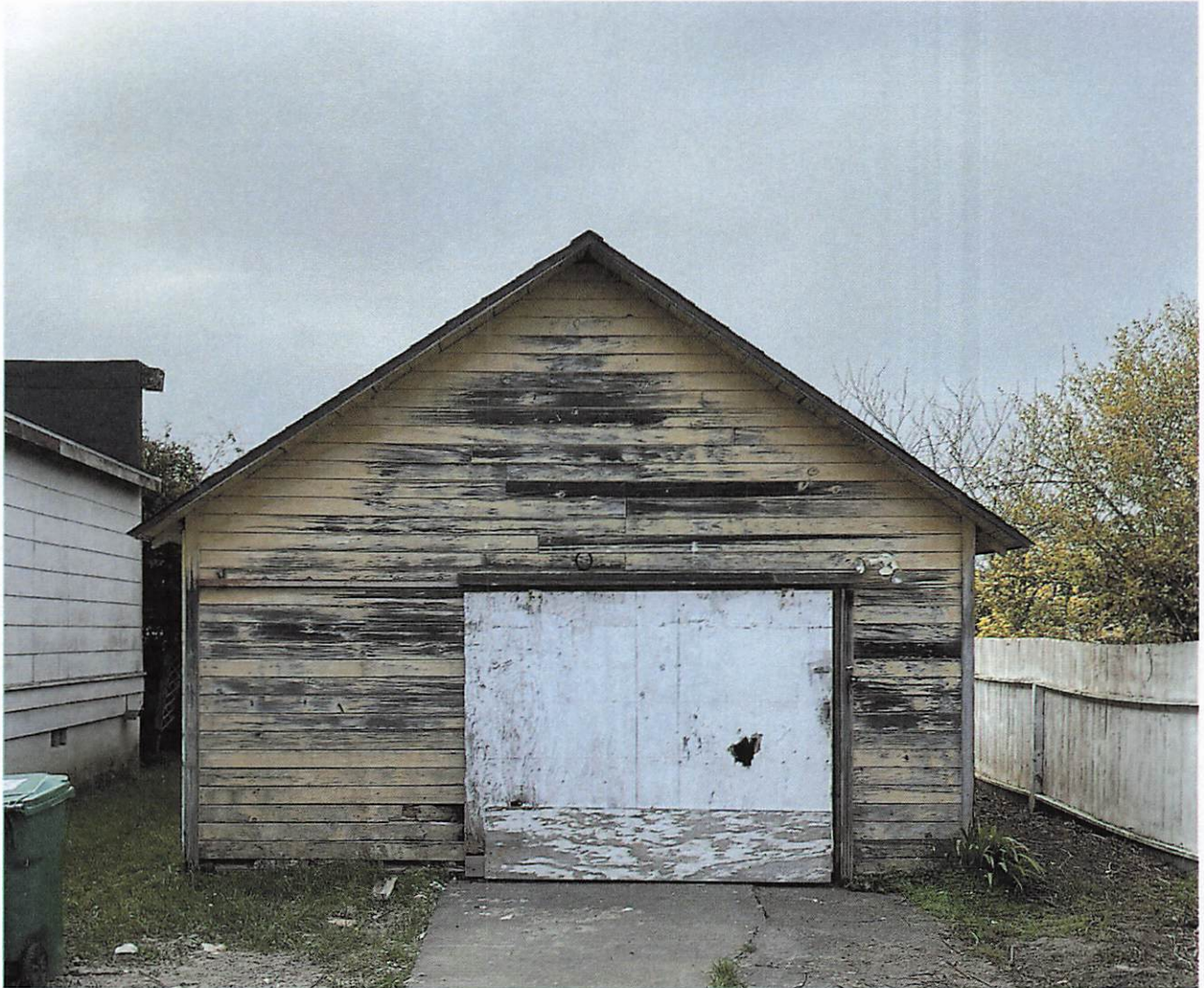
View of front (east facing) of existing garage
